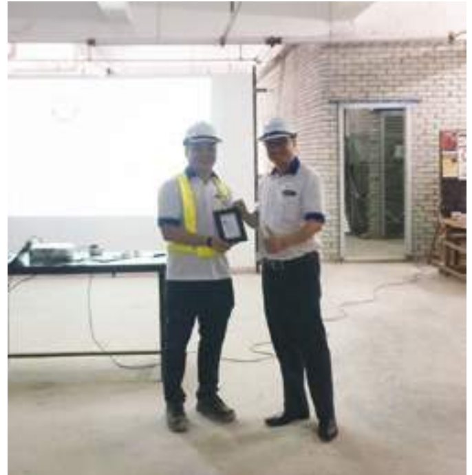
A 'No Plastic Campaign' was initiated at the Utopolis Glenmarie project location where site workers were given reusable bags and rewarded for using them
