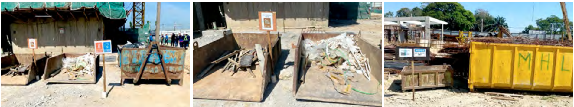
Construction waste is separated into several bins to facilitate recycling
