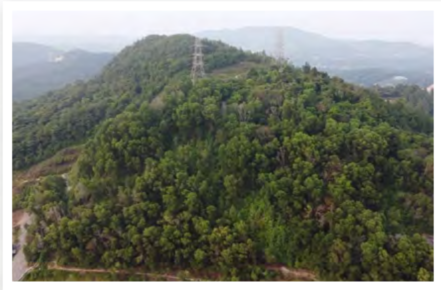
Aerial view showing the site from the west ridge side
